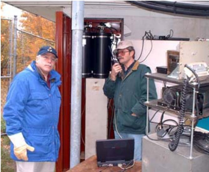
Greg KB2CQE and Bob N2CBH test the new 2 meter repeater after installation on November 2. The repeater is in the red-brown metal case, with the duplexer at the top. The old repeater can be seen on the open shelving at right.
