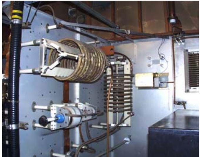
*Part of the phasor at WEVD. The phasor adjusts phase and amplitude of the RF signals fed to each antenna tower.*
