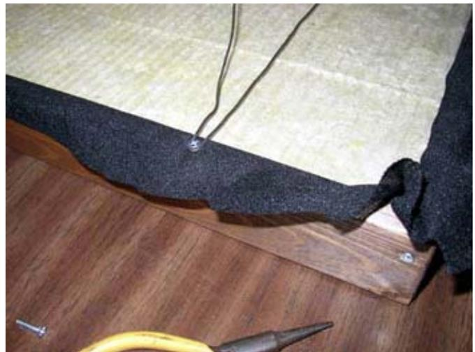
*Construction of acoustic absorption panels as designed by WB2HNA. The mineral fiber material is covered with speaker grille cloth and set in a wood frame.*
