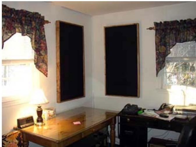
*WB2HNA's new radio room is quiet as a mouse thanks to six sound absorption panels covered in black speaker cloth.*
