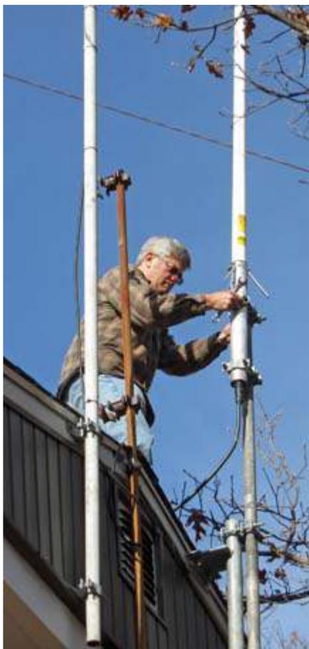
*Bob N2CBH adjusts clamps for the new UHF antenna. Old mount for the Diamond antenna is visible in the center, with support pole for 2 meters on the left.*
