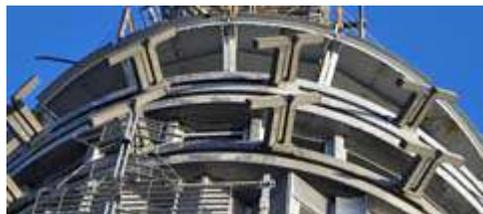
*Alford Master Antenna at Empire State Building has two rings of 16 slanted dipoles around the observation deck.*
