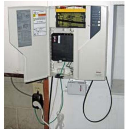
FiOS Optical Network Terminal mounted on the basement wall. (Lefthand door for access to the backup battery is open.)
