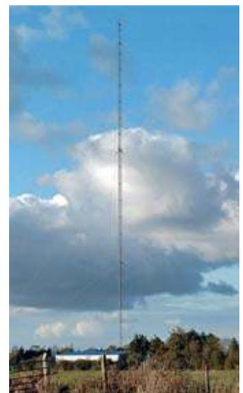
*RTÉ Radio One 252 kHz long wave transmitter site at Clarkstown, Co. Meath. The guyed mast is 813 feet tall.*
