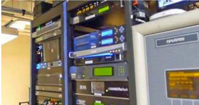
*Harris digital TV transmitter for WJLP-HD, transmitting on VHF channel 3 from 4 Times Square, New York.*
