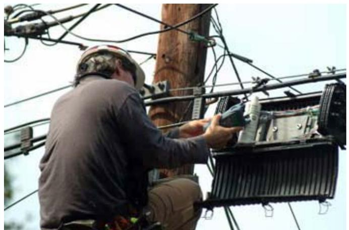
*A Verizon technician tests fiber-optic cabling at a fiber service terminal on a pole. The fiber service terminal contains equipment capable of delivering FiOS to 32 individual homes. [Verizon photo]*
