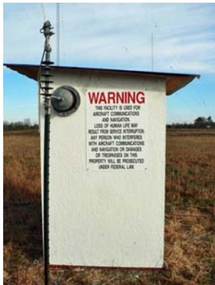
Non-directional aviation beacon **LYQ** radiates 25 watts of CW from Manchester, TN on 529 kHz. The vertical flat top antenna is suspended between a pair of 150 foot towers.
