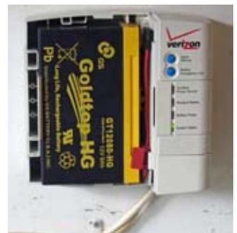
Battery backup unit for a Verizon FiOS Optical Network Terminal provides voice service backup for up to 8 hours.
