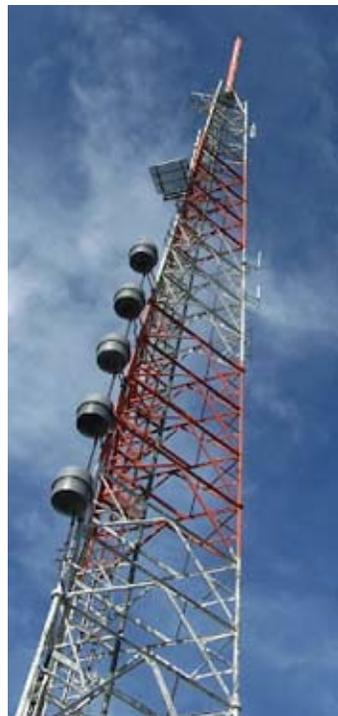
*Mt. Greylock tower, home to weather station WWF48. The barrels are radomes protecting the multi-element array for WAMC - Northeast Public Radio.*
