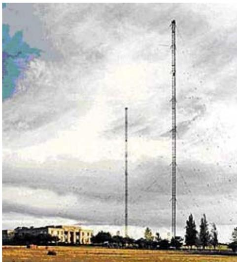
*The BBC Long Wave transmitter at Droitwich, England came on-air in 1934. Two 700 foot steel masts, 600 feet apart, hold up a wire "T" antenna for 200 kHz. It is still on-air today on 198 kHz.*
