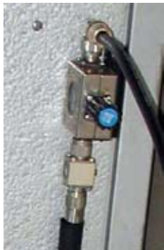
Circulator and dummy load on 2m test repeater.
