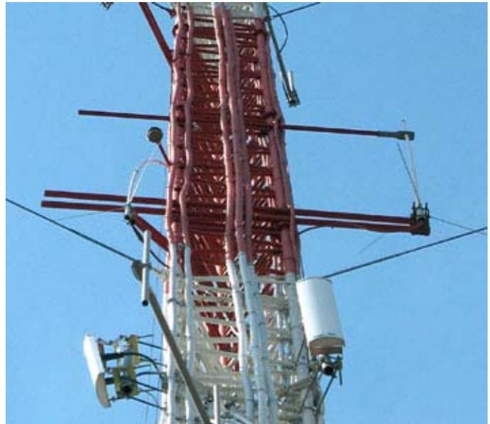
This photo, taken earlier in the year, shows the two meter repeater's antenna (middle left) trapped under a tower lighting arm. Bob N2CBH reported in July that the antenna has been freed from under the lighting arm and is now back in a vertical position.
