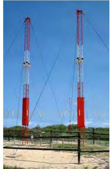
*WWVH antenna for 15 MHz has two 1/2-wave vertical dipoles positioned one 1/4-wavelength apart. The lower half of each dipole is a skirt of nine wire radials.*
