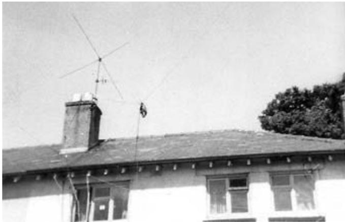
Early wire antennas were strung between the chimney and support poles in the back yard. Note the wires and feeders passing through the open shack window, far left.
