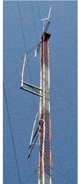
*Lake Huron ARC repeater has separate transmit antenna, top center. Receive antenna is below, slightly bent over.*
