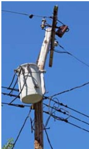
*A falling tree limb bent over this utility pole and knocked out power to WA2MCR and NM9J.*
