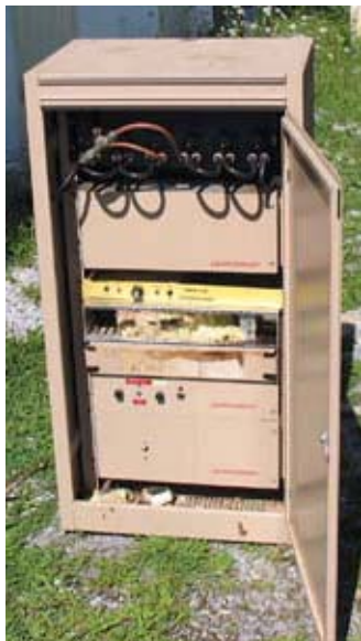
Putnam Valley 448.725 repeater cabinet with unwanted guests. See report by Bob, N2CBH starting on this page.
