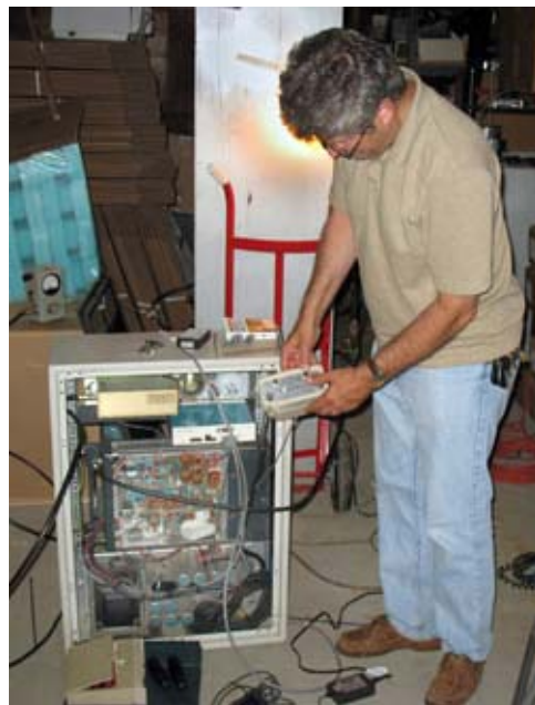
Bob, N2CBH working on the test repeater in his garage. The large cabinet behind Bob houses the six-cavity duplexer.
