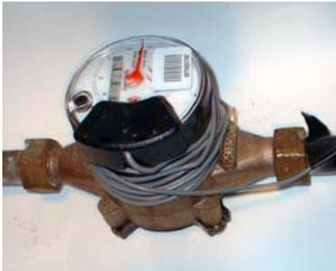
*Neptune T10 water meter. The gray cable carries meter readings to the nearby Neptune R900 Meter Interface Unit.*
