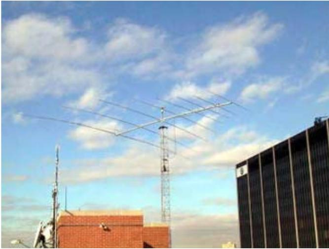
*The eight element M<sup>2</sup> log periodic used by Bob, K2TV at the CBS Broadcast Center in New York City to contact Karl N2KZ on 30 meters. This antenna covers the seven amateur bands from 40 to 10 meters. Rig is a Kenwood TS-940S.*
