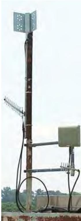
*This rooftop DAS (Distributed Antenna System) extends wireless cellphone coverage into an unserved building. [N2KZ pic.]*
