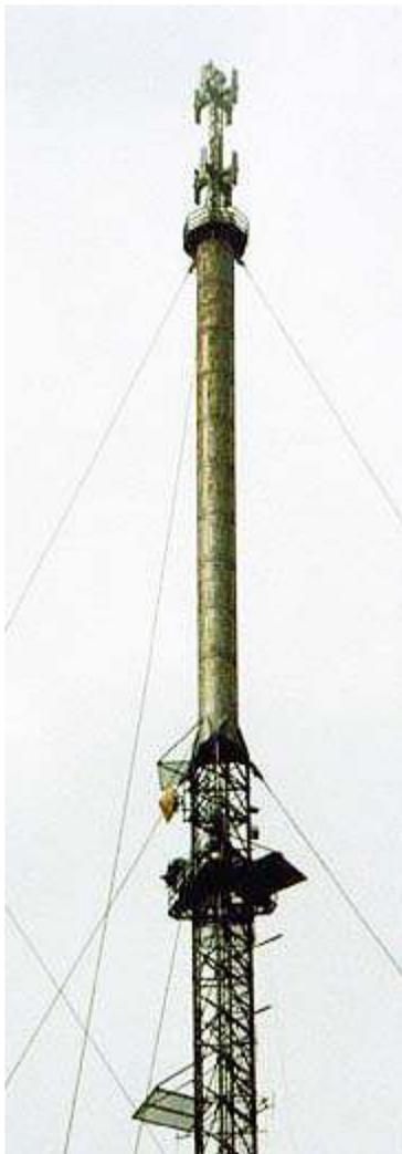
BBC Holme Moss TV and FM mast in 1984. Vertical slots for FM are just visible down the left side of the steel cylinder.
