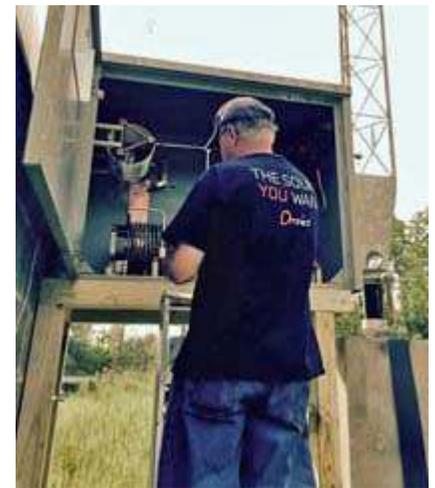
Project Engineer Tom Ray, W2TRR adjusts the coupler for the 198 ft tower in Nanuet that transmits WRCR-HD on 1700 kHz.
