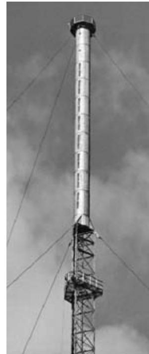
Cylindrical section of the Wrotham mast showing eight tiers of vertical slots.
