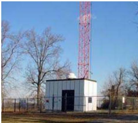
'Doghouse' at WCBS-AM and WFAN-AM transmitter site combines the output from both transmitters into one antenna.
