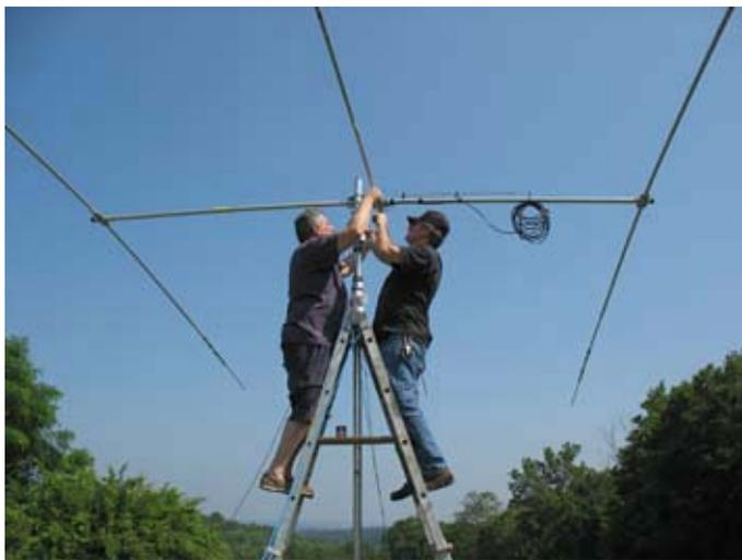
*Joe WA2MCR and Bob N2CBH busy erecting the Hy-Gain TH3Jr triband beam. Note the coil of coax fastened to the boom. After the antenna was raised into the air, it had to be lowered again to release that carefree coil of coax!*
