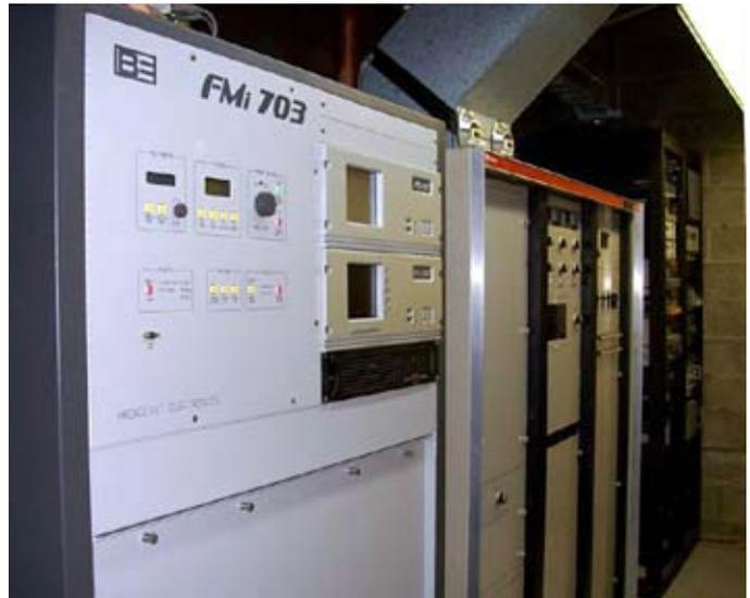
*Broadcast Electronics FMi-703 2.8kW IBOC transmitter alongside the Collins 25kW FM transmitter at WKSE.*
