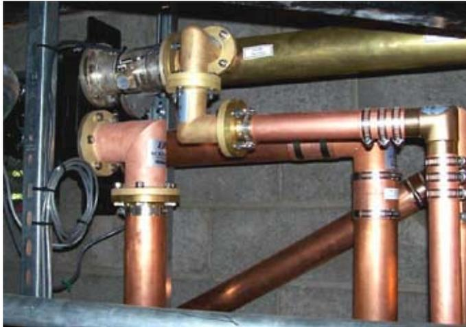
*Injector hybrid installed at WKSE, 98.5 MHz FM.*
