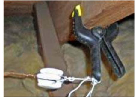
Dipole end is supported using a ceramic insulator, string and a plastic clamp in Lovji's attic. [N2CKD pic.]
