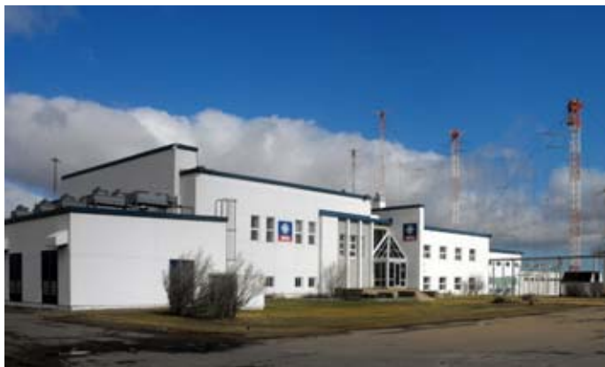
Radio Canada International TX site at Sackville, NB.
