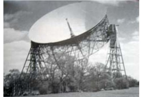
The Mark I radio telescope at Jodrell Bank had a 250 foot dish for observing the galaxies. In 1959 it tracked the Russian spacecraft *Lunik II* and in 1960 it issued command signals to the US spacecraft *Pioneer V* on its way toward an orbit around the sun.
