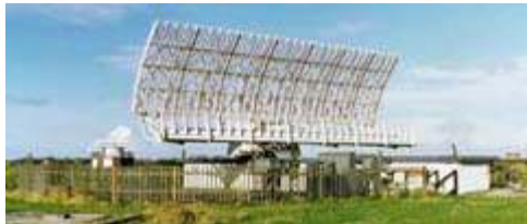
Marconi 264A 50 cm radar installation at St Annes, near Blackpool.
