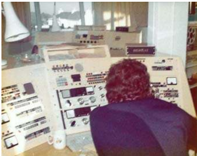
One of the operator consoles at Anglesey Radio in 1977. Note the nixie-tube digital clock on the console top right and twin Eddystone EC958 communication receivers set into the console by the operator's left shoulder.
