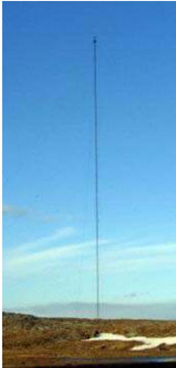
*Ingøy longwave transmitter on 153 kHz uses an 1188 ft guyed mast plus skirt radiator.*
