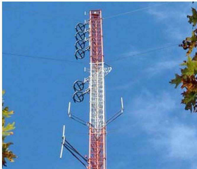
FM-stereo signal of local broadcaster WHUD is radiated from circularly polarized antennas at the top of this tower, using a power level of 50 kW ERP.
