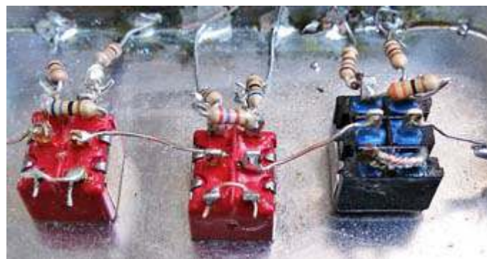
Close-up view of switch wiring. DPDT switch #1 is on the right. Resistor pi-network is wired to the terminals on the "attenuator IN" position of each DPDT switch. The switch terminals on the "attenuator OUT" side are connected together with a wire link. The tinfoil case can be readily soldered for a chassis ground connection. [N2CKD pic.]
