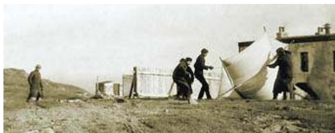
Guglielmo Marconi (left) watches as his helpers prepare to fly a large kite from Signal Hill, St. John's, Newfoundland in December 1901. The kite would support an antenna for reception of transatlantic signals.
