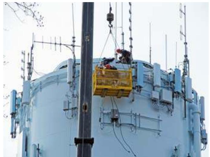
Antenna workers make adjustments on the NE side of Benefield Boulevard water tank. Note the dangling hardline below the basket.
