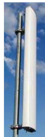
Cell-site antennas require radomes.
