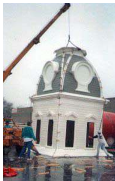
Fiberglass cupola could provide a stealthy antenna site.
