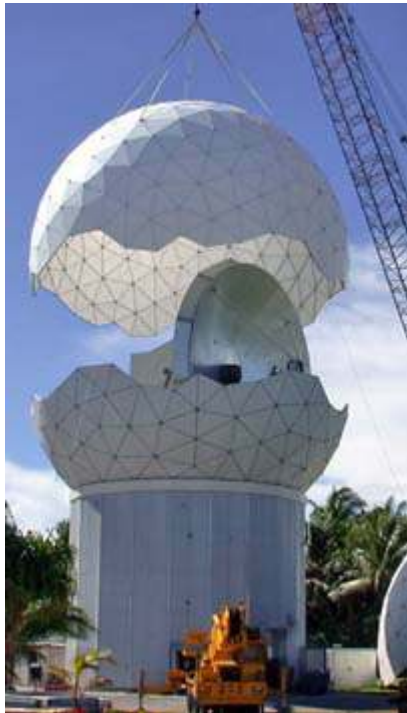
Assembly of a 68 ft Essco radome, with steerable radar dish inside.
