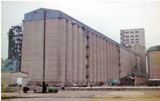
*Seaforth Grain Terminal. Storage silos are in the foreground with 300 foot tower building at rear right.*
