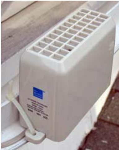
Rain sensor mounted on horizontal bar.
