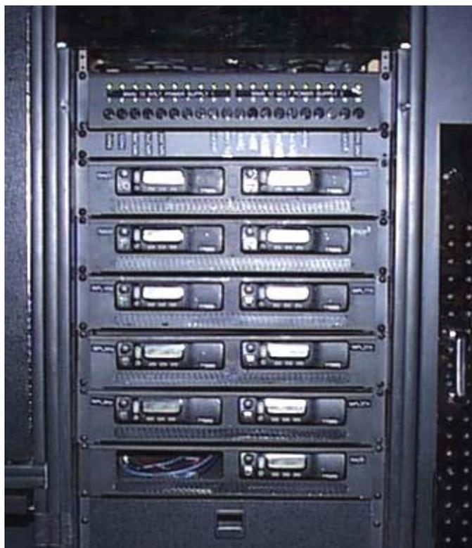
Rack-mounted Motorola mobile radios used for studio coordination at MTV Networks.
