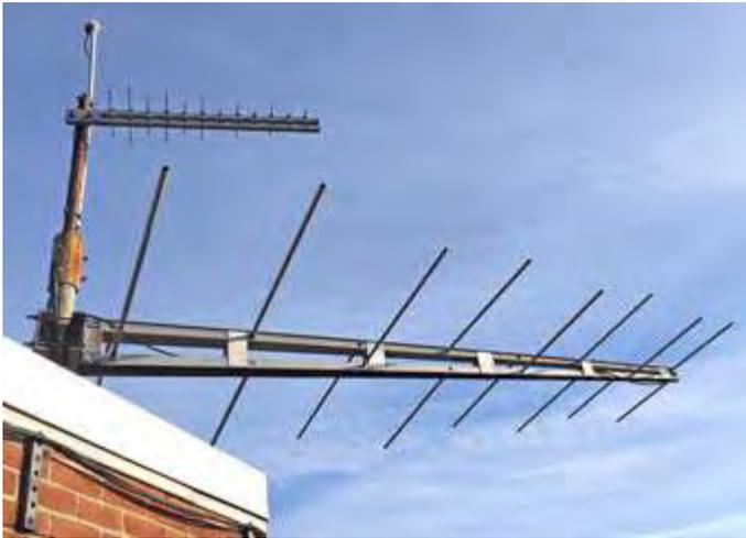
*Quadrade Channeler Log-Periodic single antennas, series QCA at Karl's workplace. UHF (top) and low-VHF below.*
