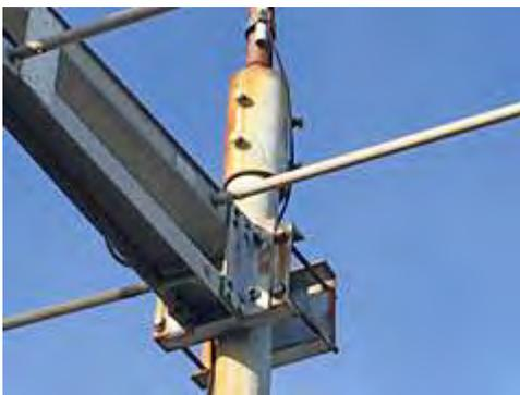
*Substantial mounting hardware for Quadrade Channeler single VHF antenna.*
