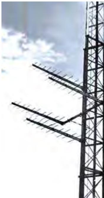
Scientific Atlanta **Quadrate Channeler** antenna array for CATV, side-mounted on a tower. Four log-periodic antennas are arranged in a diamond pattern.
