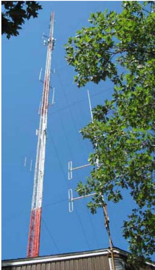
*Antennas at the 449.925 repeater site. Folded dipoles are for 2 meter standby repeater; vertical colinear is for the 449.925 KB2CQE repeater.*
