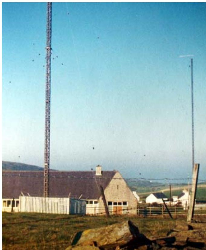
Post Office Coast Station “Anglesey Radio”, **GLV**, stands at the entrance to Liverpool Bay. Twin masts, pictured in 1977, supported a vertical T-antenna for 500 kHz transmissions.
