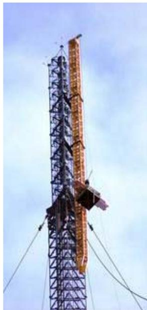
*By early December, all sections of the new VHF-FM antenna were in place at the top of the 2000 ft tower. (The yellow structure alongside is the gin pole, used to swing sections into position.)*
