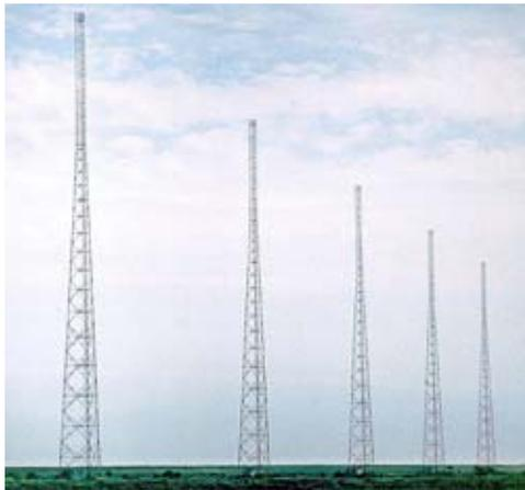
*BBC World Service transmits to Western Europe from Orfordness, England using this five tower array on 648 kHz.*
