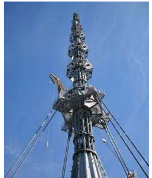
The 408 foot spire atop One World Trade Center is held in place by eight HPTG-I high-performance tower guy assemblies from Phillystran.
