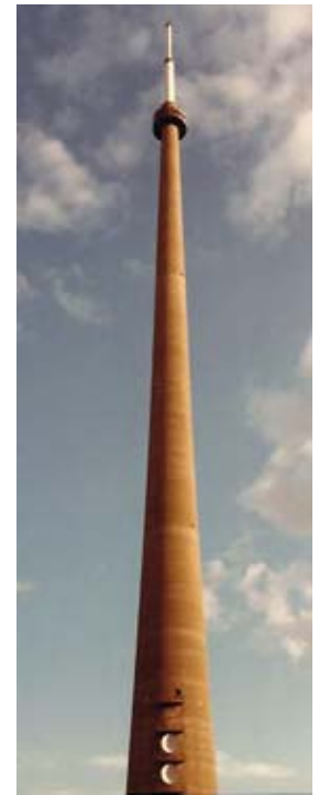
Emley Moor TV transmitter site in Yorkshire has a 1084 foot concrete tower.
