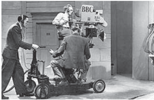
EMI's television system was all-electronic with mobile cameras.
