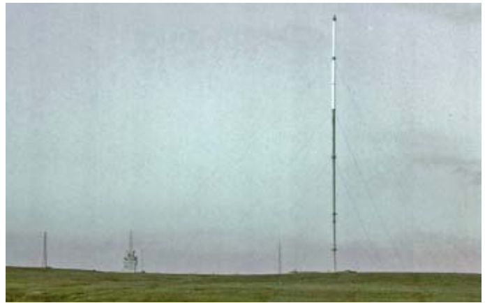
"New" 1015 ft tubular steel mast at Winter Hill is at right. The white sections on top are fiberglass shrouds for the UHF and VHF TV antennas. Shorter masts at left were used for Post Office microwave links and police/fire radio.
