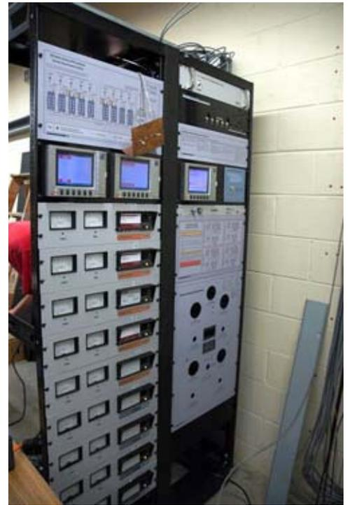
*Monitor and Control system installed by Broadcast Devices Inc. to keep track of the nine separate stations at Senior Road.*
